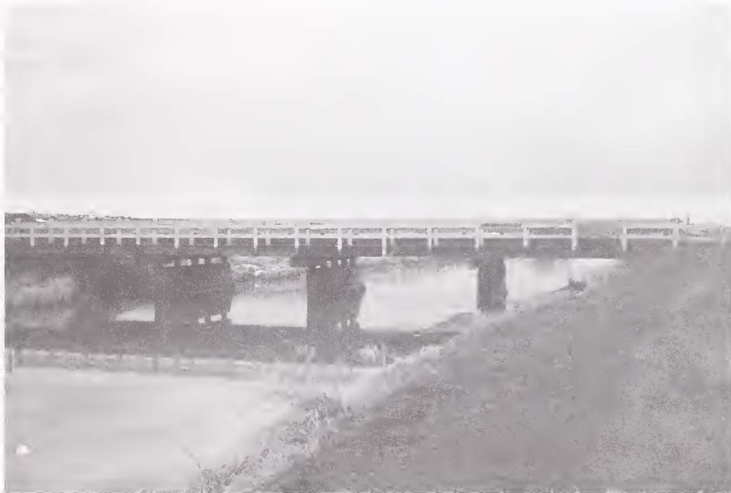
Dodson South Canal Bridge in Malta. Note the sidewalk, laminated wood sheathing that protects the pile bents.
